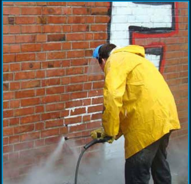
INTELblast and partners are offering a wide range of industrial cleaning services that requires a high level of know-how, experience and technology. We have specialized in blasting technologies involving lava, granite, dry ice, ultra high pressure water blasting and ductwork cleaning.
